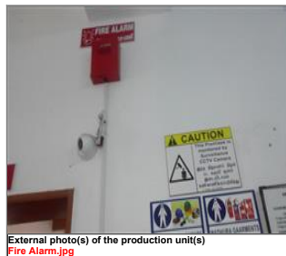
External photo(s) of the production unit(s) Fire Alarm MCP.jpg
